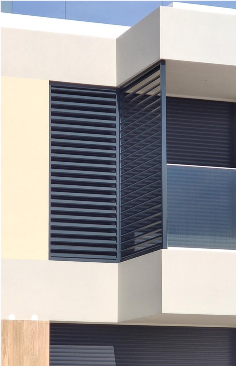
Photo of a villa in the same housing estate
